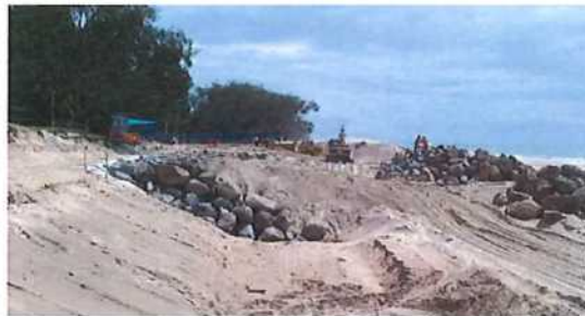
Figure 6.5: Buried Seawall under construction (GCCC 2016)
