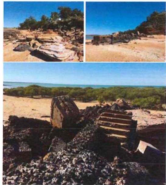
Figure 3.4: Shoreline protection in front of Roebuck Bay Caravan Park, Town Beach. Upper left: Mix of native and placed rock in the foreshore at base of cliff. Upper right and lower: groyne structure at midpoint of caravan park frontage made of old building material.
