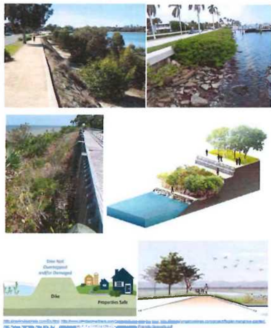
Figure 6.17: Adaptation examples. Sloping seawall (upper left), vertical seawall with mangrove planter at base (upper right), feature walkways (middle), levy / dike structures (lower)
