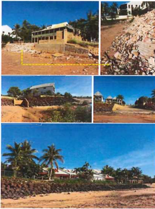
Figure 3.3: Shoreline protection in front of Catalina's, Town Beach
