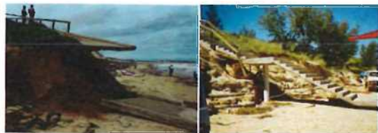
Figure 6.2: Cable Beach post TC Rosita 2000 showing (left) undermined beach access ramp and (right) beach access stairs (photo source: Shire of Broome, JCU 2000)
