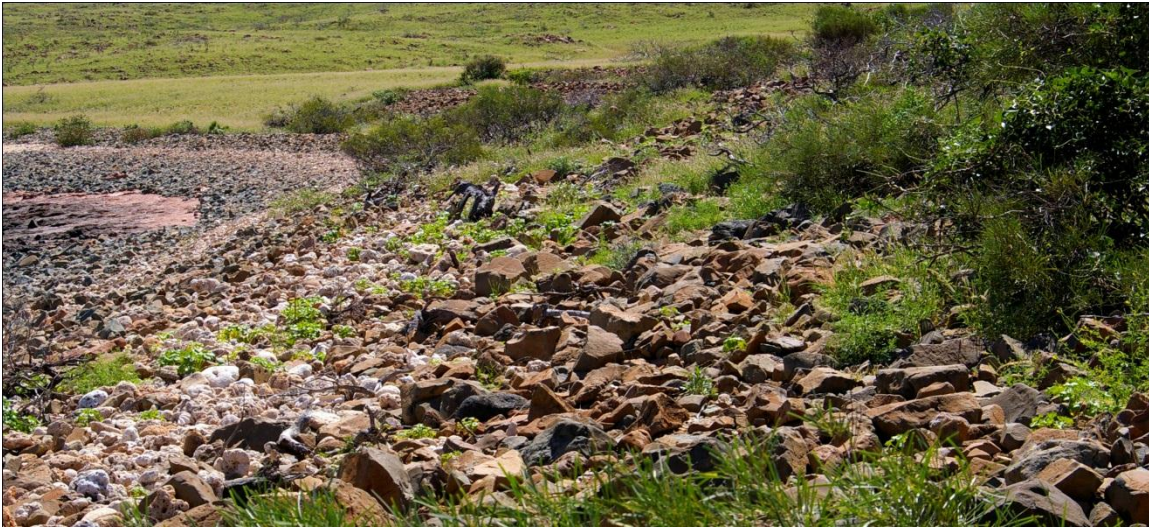
Figure 7: The bund facing the southern channel side, viewed facing west
